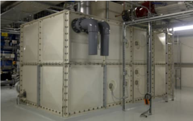
Figure M09: Typical cold water storage tank
